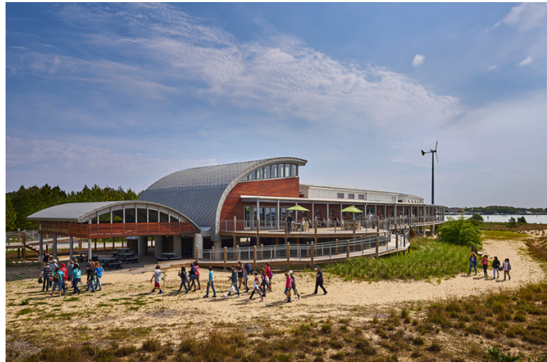
The Brock Environmental Center in Virginia Beach, Va., was projected at a 15.5 EUI, but performed in its first full year of measurement at 14.12 EUI. Image Courtesy: Prakash Patel/SmithGroup JJR.
